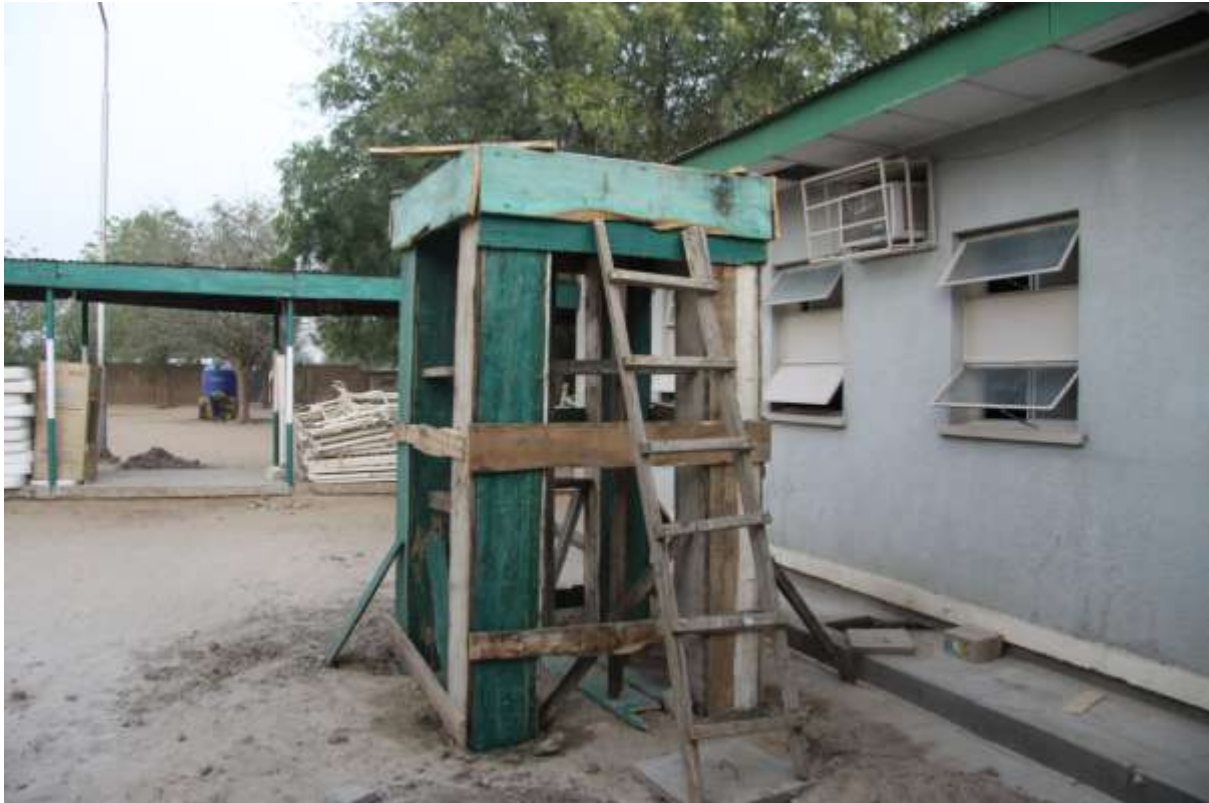
Picture 3: Overhead booster tank structure erected on team's advice
